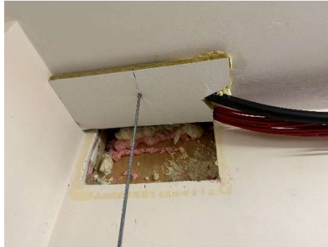
Figure 02 The fire foam that is not tested for that location
