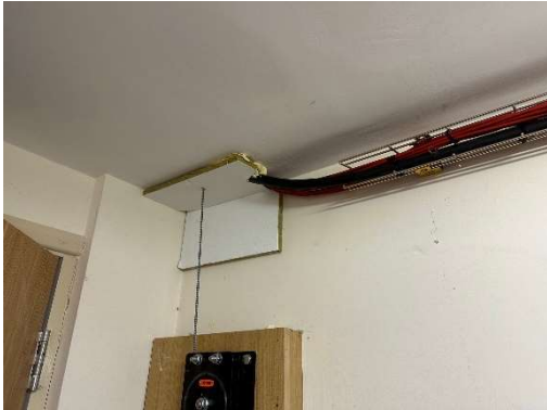
Figure 01 The location of poor fire compartmentation in the theatre
