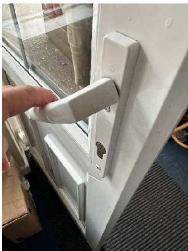
Figure 05 The fire exit without a thumbturn on the inside
