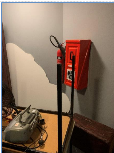
Figure 01 – Blocked fire extinguisher onstage in the theatre
