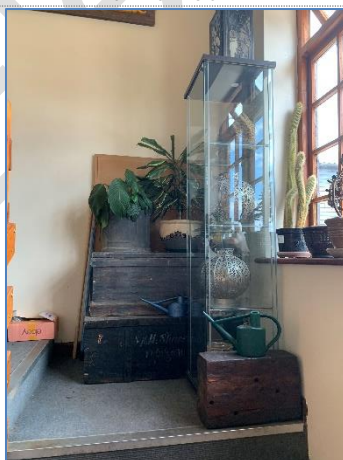
Figure 03 – Items on the means of escape stairs from the Estates manager’s flat
